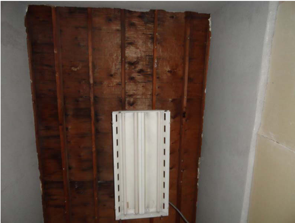
North elevation facing south
