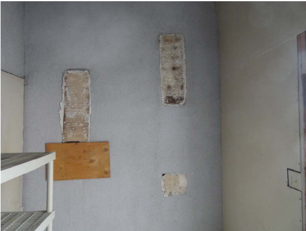
South elevation facing north
